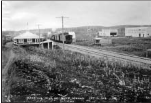
Wasilla was little more than a small depot back in 1918 when this photo was taken. We're proud to support growth and construction in Alaska's railbelt communities.
