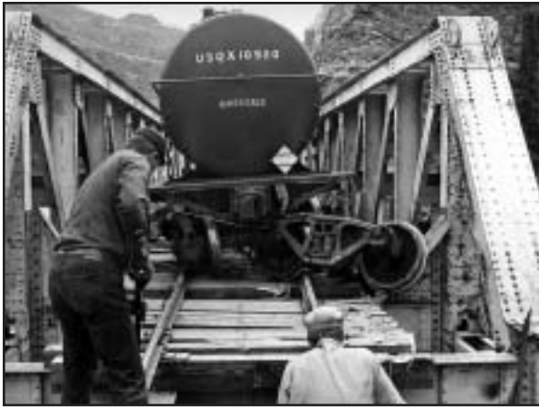
Upgrades in our line mean that track-caused derailments are a fraction of what they were a decade ago.
