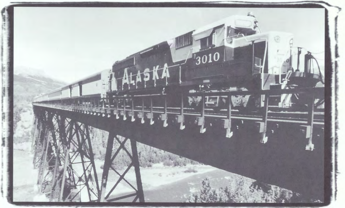
Southbound passenger train crossing Riley Creek near Denali Park Depot. Photo by Clark Mishler
