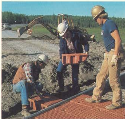
Maintenance workers installed a new, high technology material at railroad crossings that will provide a better crossing surface for the traveling public.
