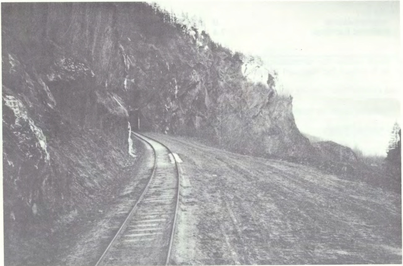
Mile 52.5 after removal of fault damaged tunnel by 32,000 pounds of explosives. (Photo by Bill Coghill)
